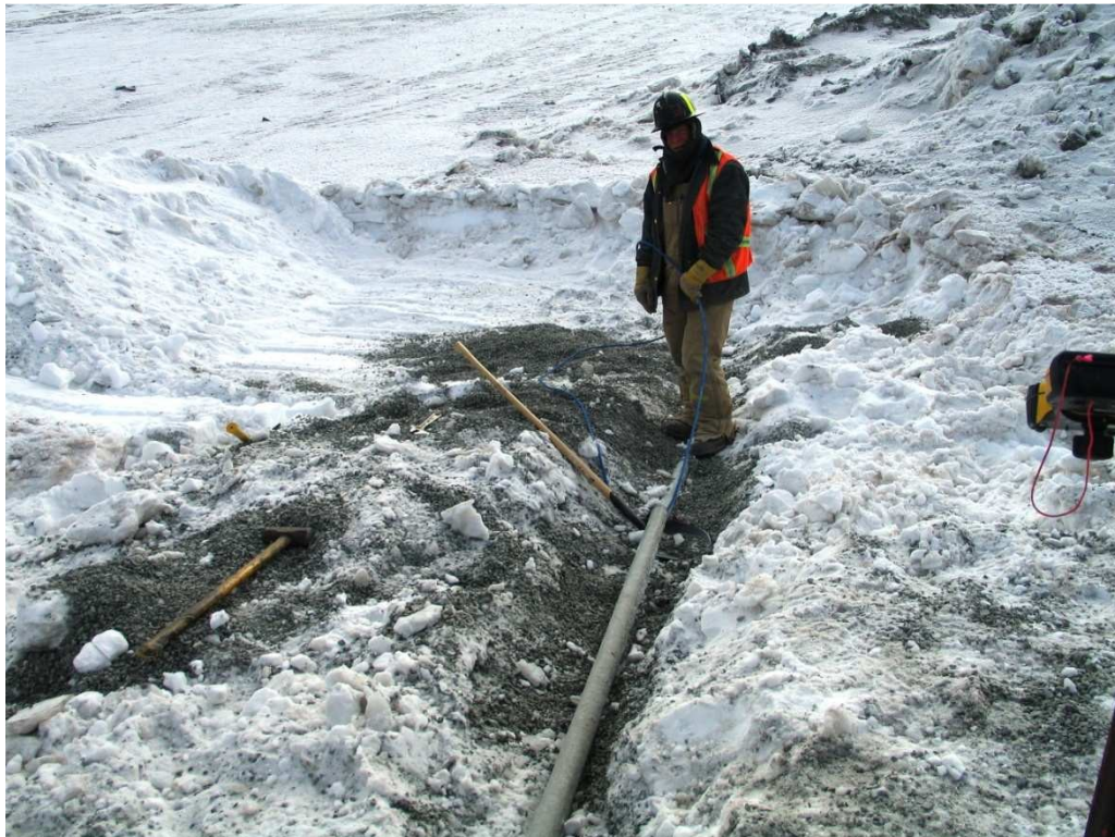
Photo 7: Two pipes separated. Cable is being pulled through the top pipe Sta 0+85 us.
