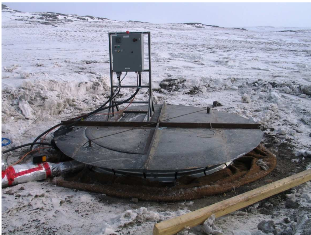
Photo 2: Electrical panel in place sump 2..
