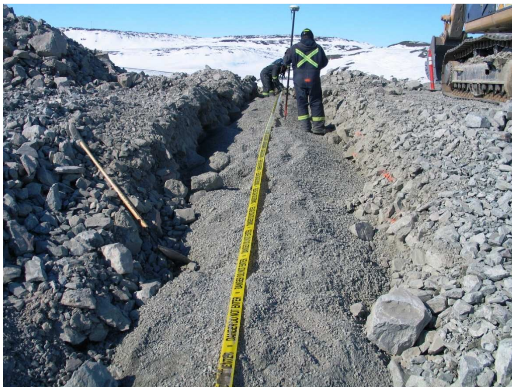
Photo 5: Final crush across the top of the dam Sta 1+30 us
