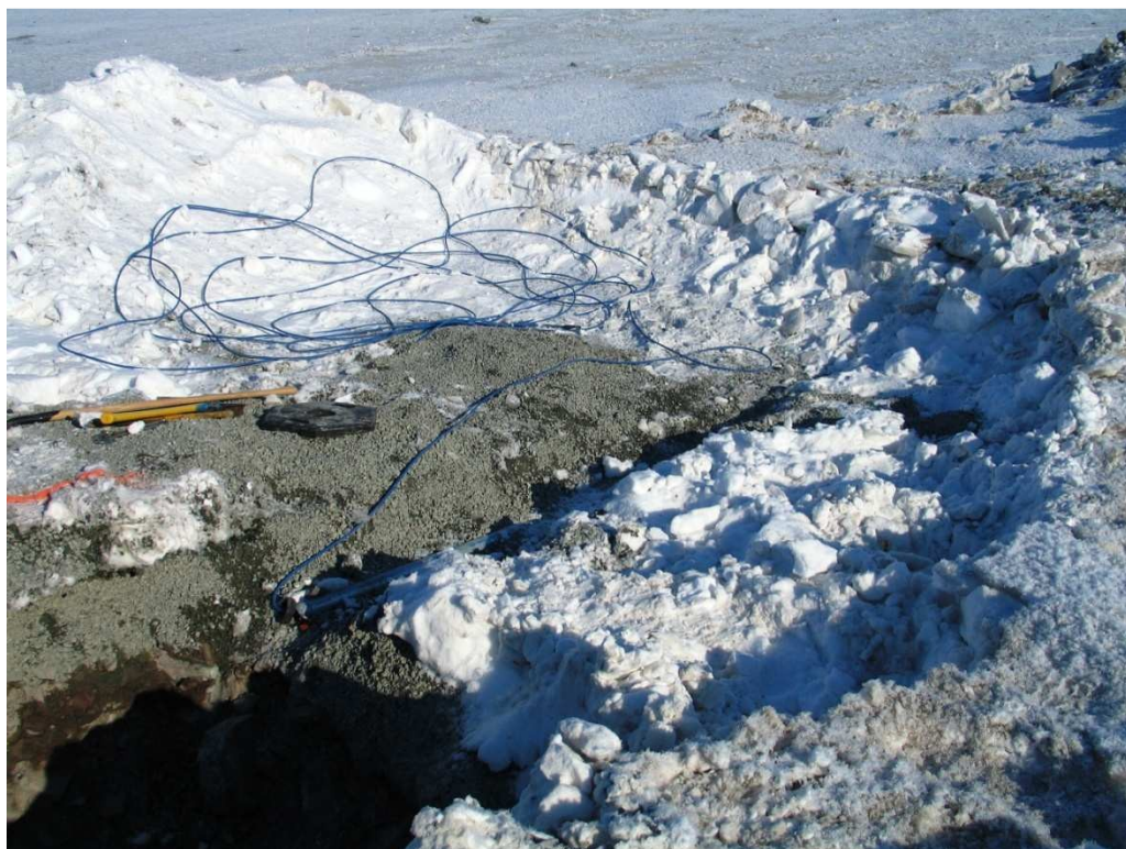
Photo 7: Two pipes separated. Cable is being pulled through the top pipe Sta 0+85 us.
