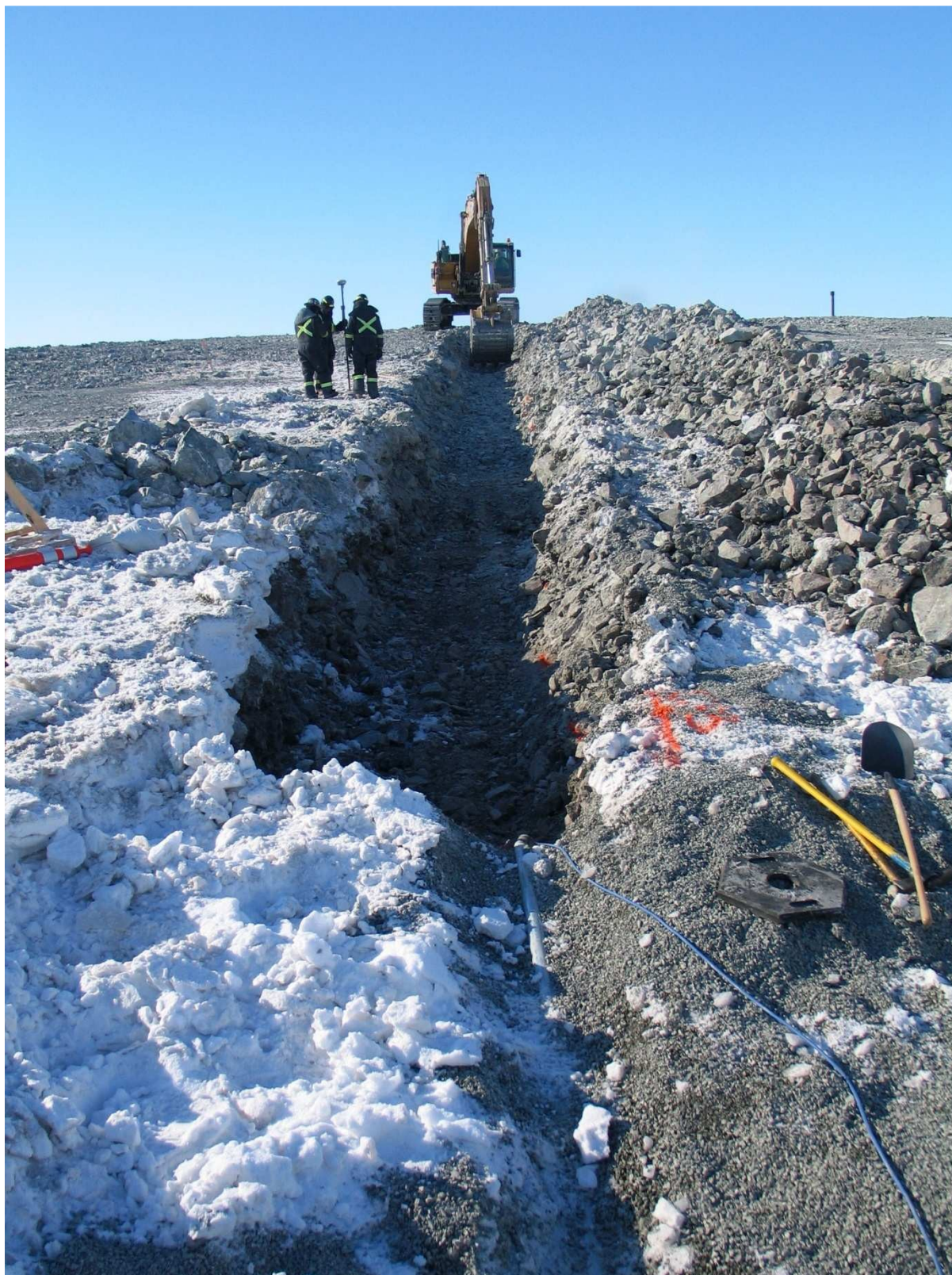
Photo 9: Excavation at Sta 0+85 us. The red paint line indicates where the underground line is located. At the pipe it was ~ 1m down
